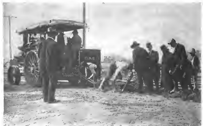
Breaking Ground for Road Improvement Outside Detroit.
